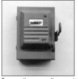
Be sure the power disconnect switch is in the on position.
