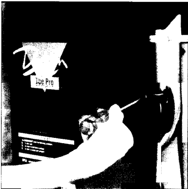
Figure 15 — Opening main panel.
