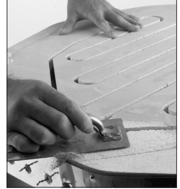
Sand the peeled areas of the lid and reapply the coating.
