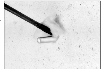
If the hole is 1/2" in diameter, stuff ceramic fiber around the protection tube.
