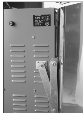
The hinged switch box has a support arm on the side.
