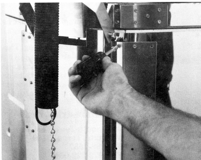
Installing the back support plate.
