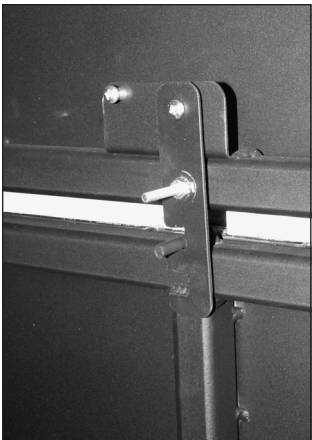
The swing-away vent latch in the closed position
