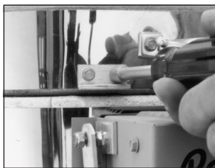
Installing the Prop-R-Vent latch onto the new lid.
