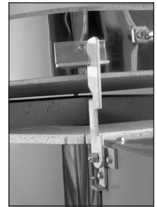
The Prop-R-Vent is shown here in the extended position.
