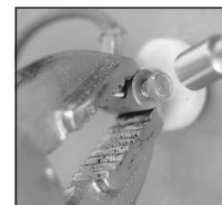
Installing the element connectors.
