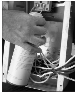
Cleaning the switch box with canned air.
