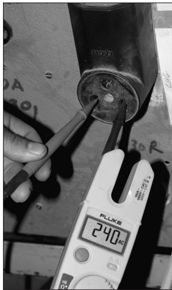
Checking the voltage of a wall outlet in the Paragon factory.
