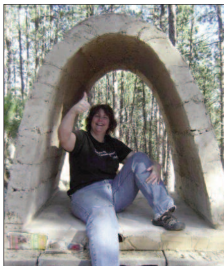
The completed castable refractory arch.
