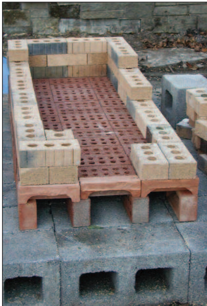
Here you can see the 3 channels which are the primary air entries in this design. The channels extend right through to the other end to provide enough for full combustion (see the notes on proportions at the end of this section). During firing, one or more entries can be closed at either end to help vary the atmosphere inside.
