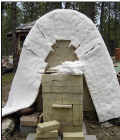
The fiber is easily cut and shaped.
