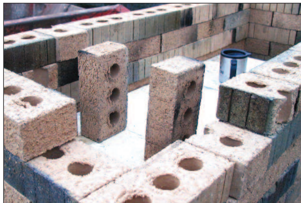
If possible, use pre-fired bricks as your support bricks.
