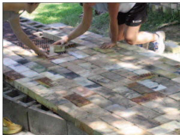
First layer of hard brick. Note the expanded metal base.
