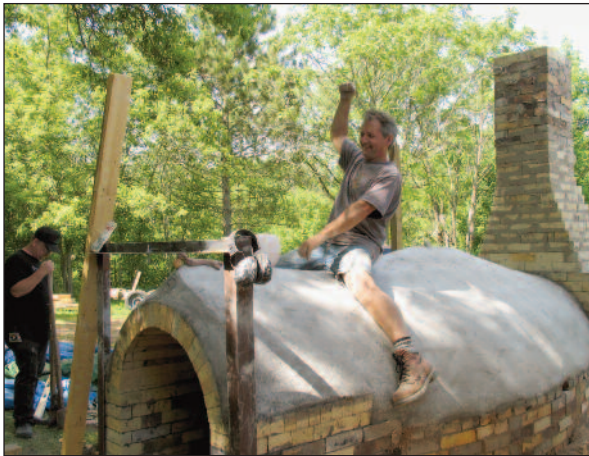
The kiln is almost done. Three coats of castable. The stack is done.
