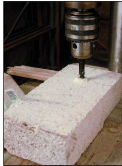
Make sure you use a masonry bit to drill the holes.
