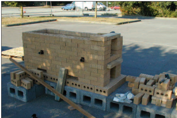
In this picture you can see the mouseholes on one side and the primary air entry at the front.
