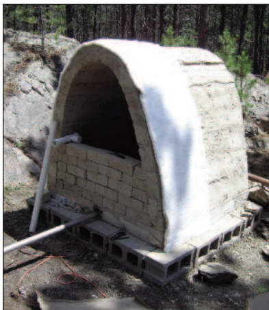
A one-inch layer of 2600° ceramic fiber.
