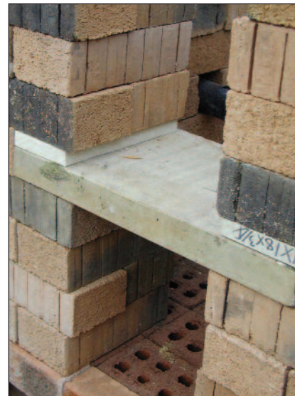
The upper hole here is for stoking. The lintel is made from thick kiln shelf. I have used cast firebrick pieces before, but they lack strength and are short-lived.
