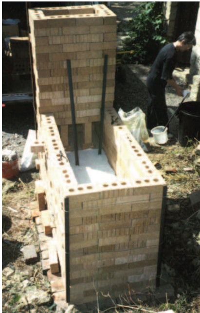
Chimney height is adjustable during firing.
