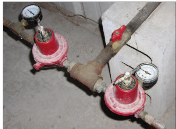
Reg can regulate his propane gas pressure as it enters his car kiln.
