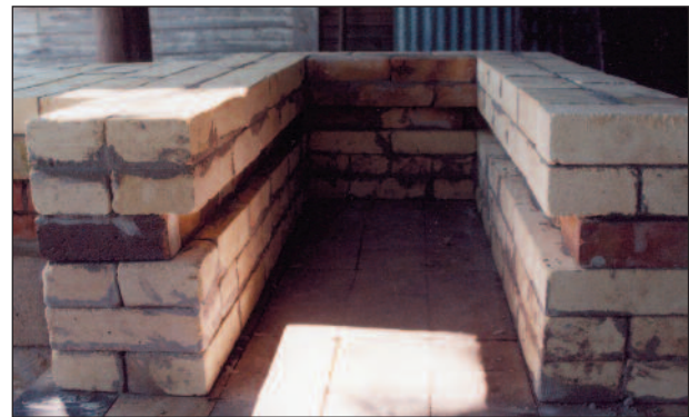
Looking into a completed firebox.
