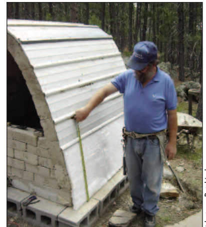
Steel protects the fiber and brick.
