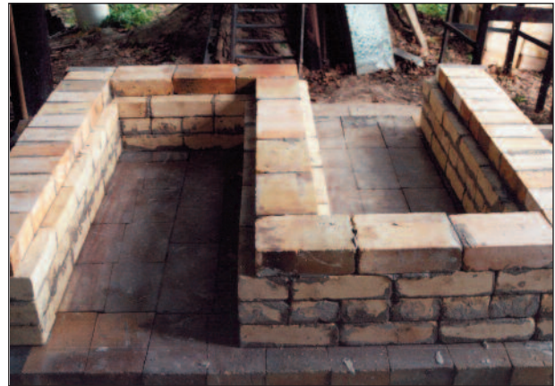
The first four courses of the fireboxes mortared in place. The fourth course is built with 6" X 9" bricks, to create the ledge for holding the fire grates in place.
