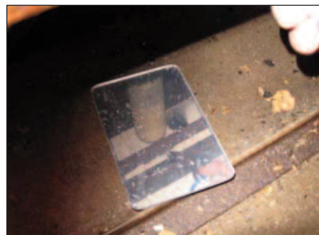
Lighting the pilot using a mirror.
