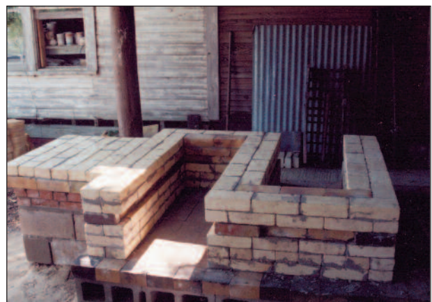
The chimney floor and completed fireboxes.
