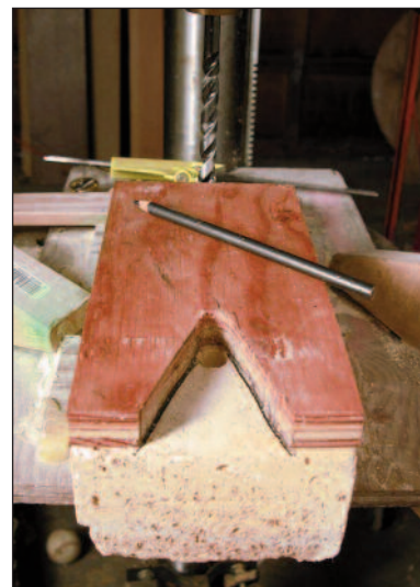
The widest part of the triangle is as wide as the angle iron used on the roof.
